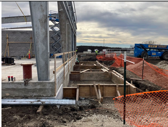
Concrete form work was in place for the Greensand Filter Foundation Pads on the west side of the building.
