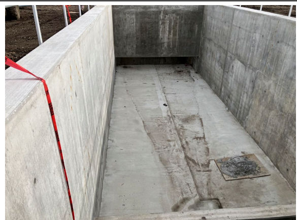
Interior of the backwash waste settling tank.
