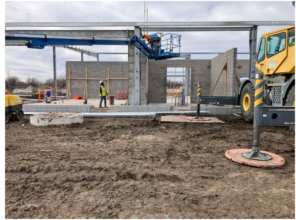
The interior masonry block walls for the various rooms had been constructed.
